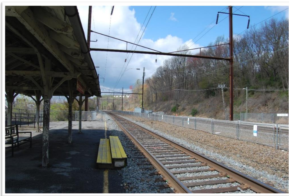
Exhibit 17. Photo of Historic Station track side accommodations (April 2022)
